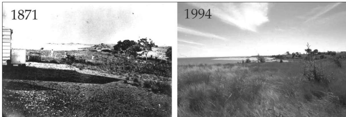
Figure 4. Identical views from the Customs House, looking north-east, over what George Phillips described in 1866 as 'open country'. (1871 photograph, Captain Sweet, courtesy of the John Oxley Library neg no. 67334; 1994 photograph, Brett Stubbs).
